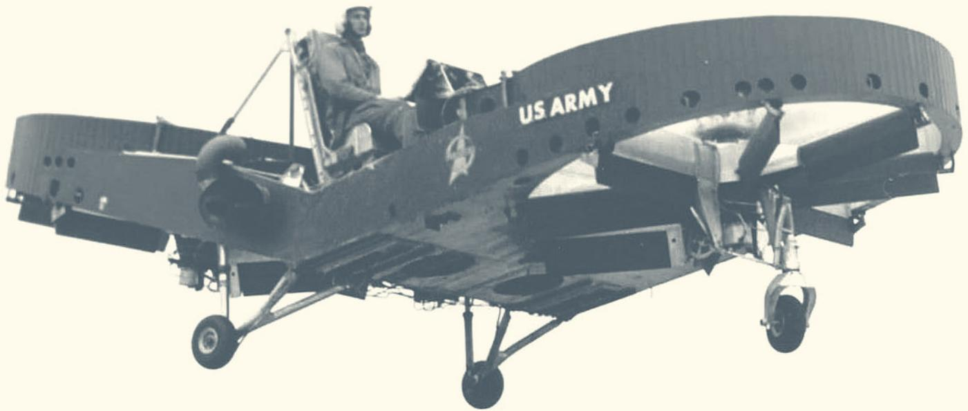
the AirGeep was primarily envisioned to operate only a few feet above the ground. Empty weight of the AirGeep at this time was 1,848 lb, with a maximum takeoff weight of 2,350 lb.
